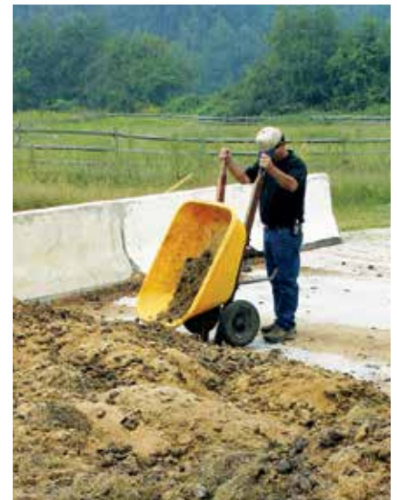
Manure storage structure with Jersey walls and concrete floor.
