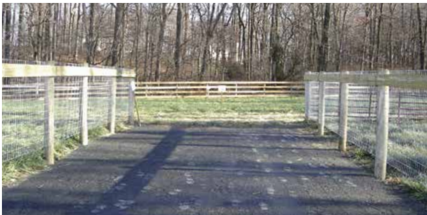
Completed heavy use pad.
